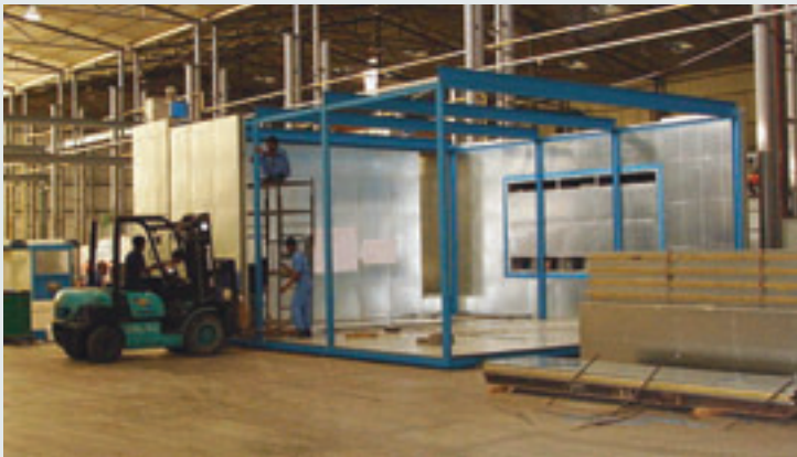
Oven under constuction
